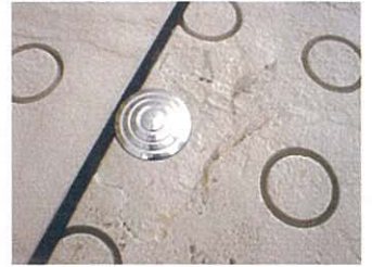
TACTILE MARKER INSTALL ON GLASS MATERIAL BY BOLT-LINE WITH ADHESIVE METHOD NO ANY DAMAGE
